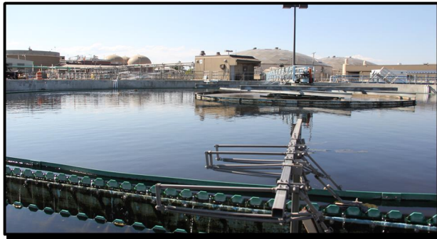
The Yakima plant processes wastewater from homes and businesses in Yakima, Union Gap, Terrace Heights, and Moxee.
