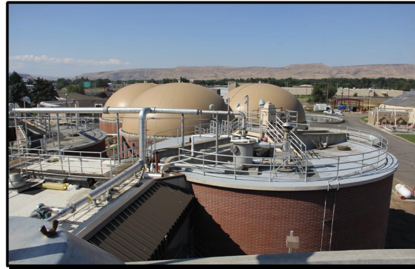
The Yakima Regional Wastewater Treatment Plant has won the 2014 DOE Outstanding Performance Award.
