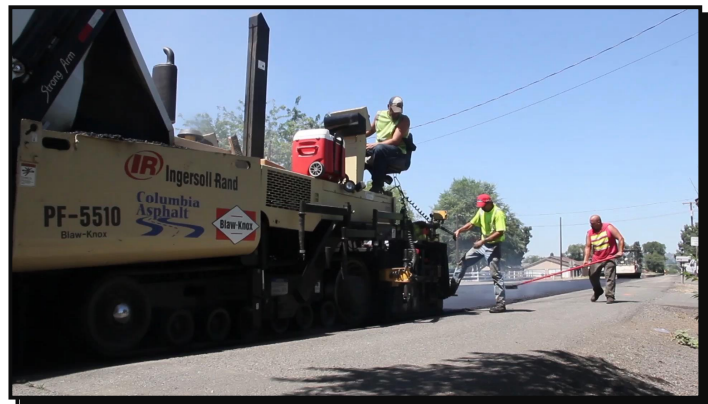
Crews from Columbia Asphalt work on a section of the nearly 120 lane miles of roads in Yakima that have been repaved in the last two years.
