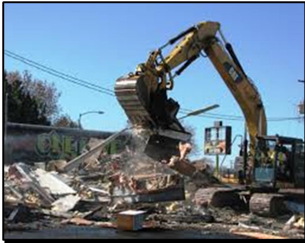
Crews demolish a former Tiger Bin Mini-Mart at the corner of Nob Hill Boulevard and 24 th Avenue on March 9 th .
