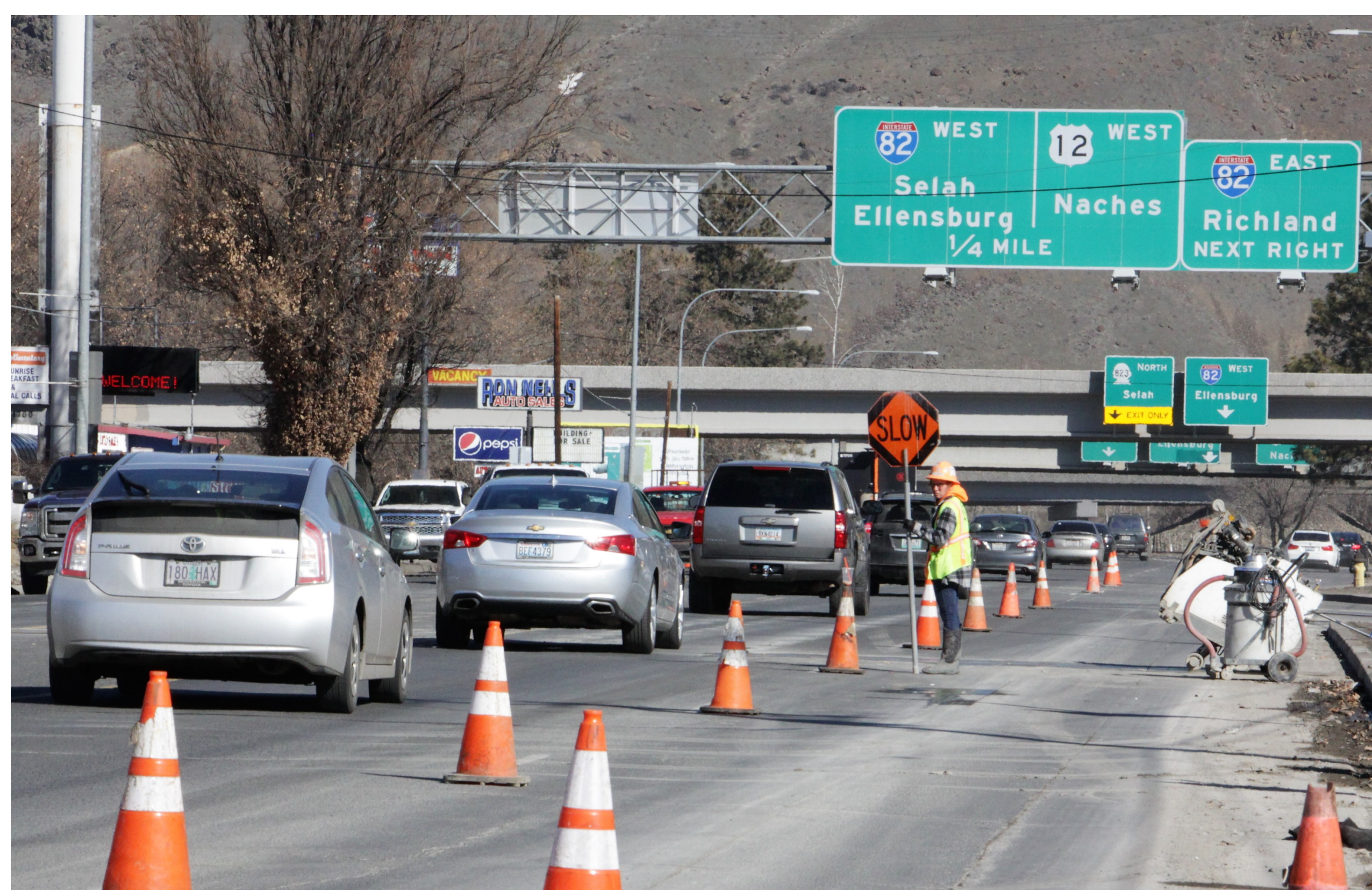
A flagger directs traffic as crews begin on Phase 1.
