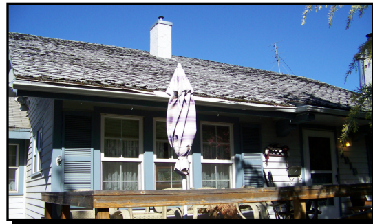
This Yakima home had several issues including a falling roof and peeling paint.
