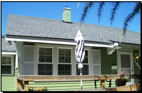
Through the ONDS Emergency Home Repair Program, a new roof was installed and the home was repainted at no cost to the owner.
