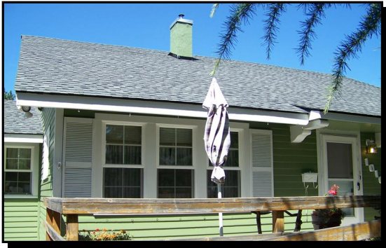
Through the ONDS Emergency Home Repair Program, a new roof was installed and the home was repainted at no cost to the owner.
