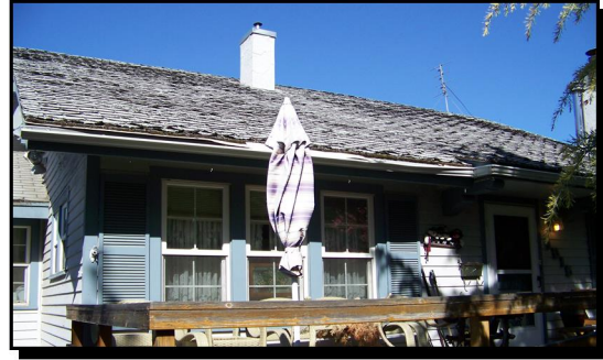
This Yakima home had several issues including a failing roof and peeling paint.
