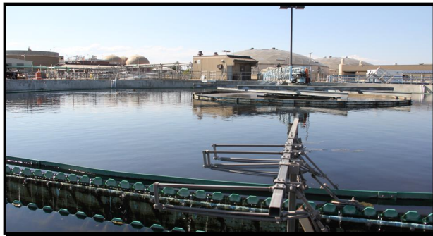
The Yakima plant processes wastewater from homes and businesses in Yakima, Union Gap, Terrace Heights, and Moxee.
