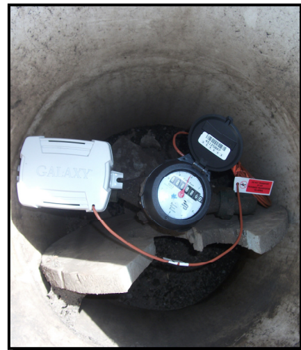
New water meters are being installed in Yakima to improve both efficiency and accuracy.
