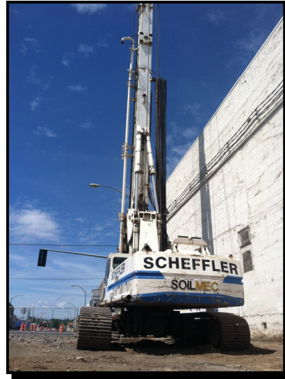
A continuous flight auger will drill retaining wall shafts and fill them with concrete.
