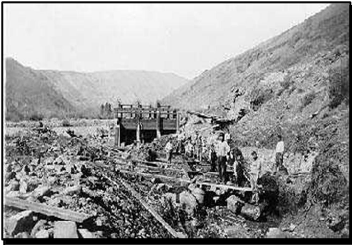
This undated photograph shows ongoing construction of an early irrigation canal in the Yakima Valley. Today, water is delivered by such canals to more than 460,000 acres of land in the region. Irrigation has been the key to making the Yakima Valley one of the most productive agricultural regions in the world.
