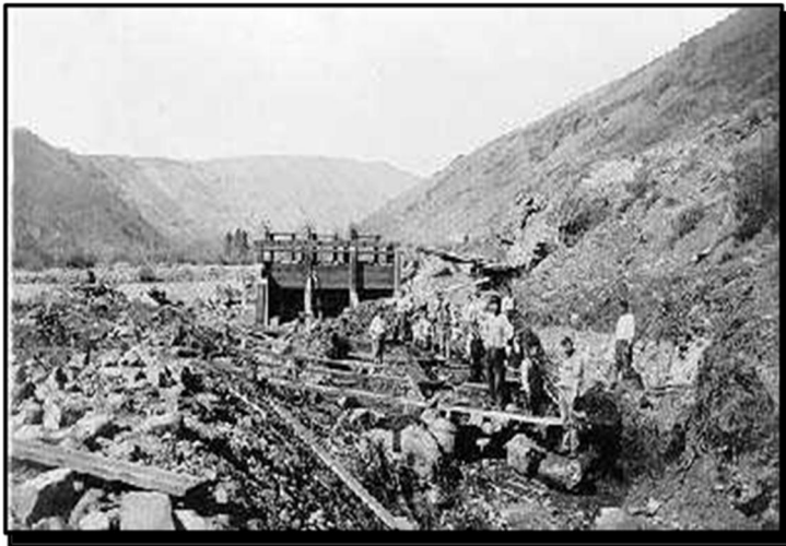
This undated photograph shows ongoing construction of an early irrigation canal in the Yakima Valley. Today, water is delivered by such canals to more than 460,000 acres of land in the region. Irrigation has been the key to making the Yakima Valley one of the most productive agricultural regions in the world.
