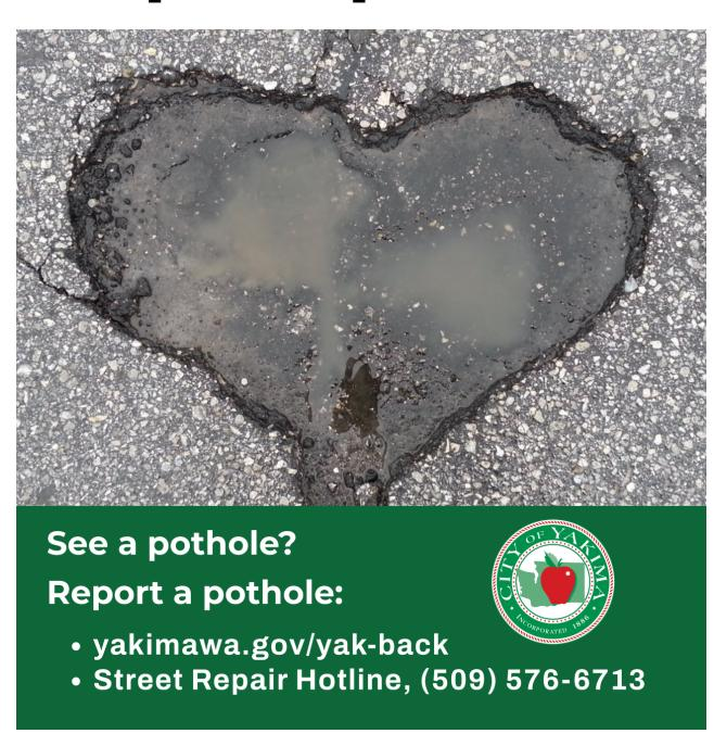
Potholes are not uncommon this time of the year due to the "freeze-thaw cycle" Yakima experiences when precipitation, in the form of rain and/or snow, seeps into small cracks within the asphalt pavement.
