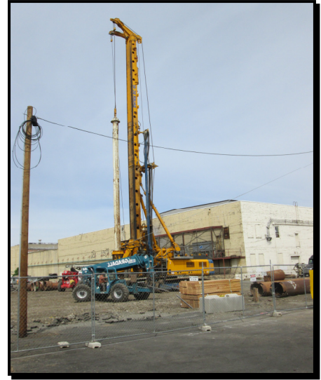
A 70-foot tall drilling rig towers over the MLK, Jr. Blvd underpass construction site.
