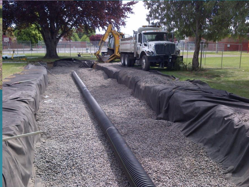
Spray Park Drain Field - 2012
