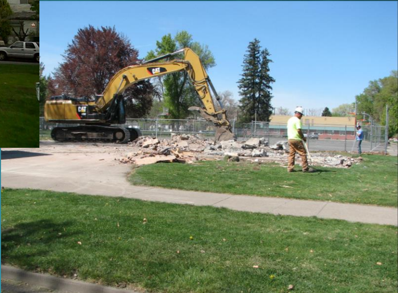
Old Bath House Removal - 2016
