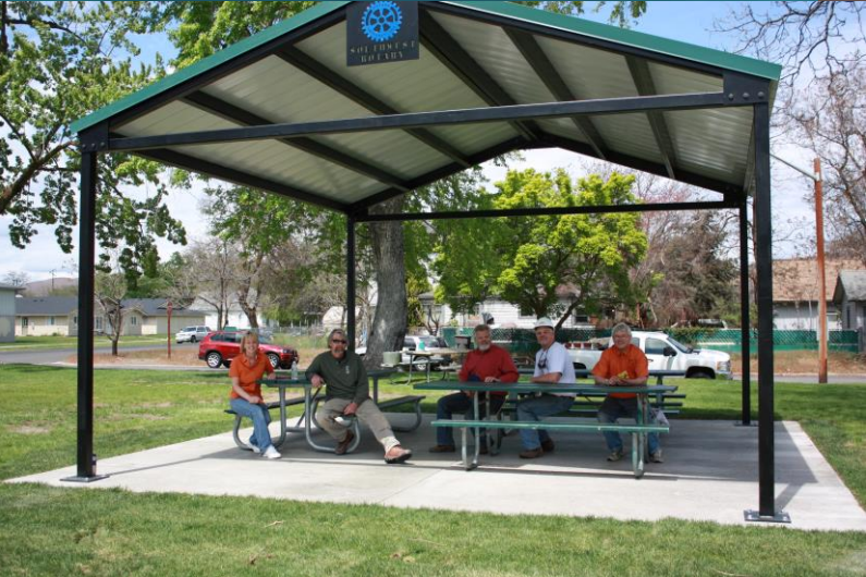
Existing Rotary Picnic Shelter - 2012
