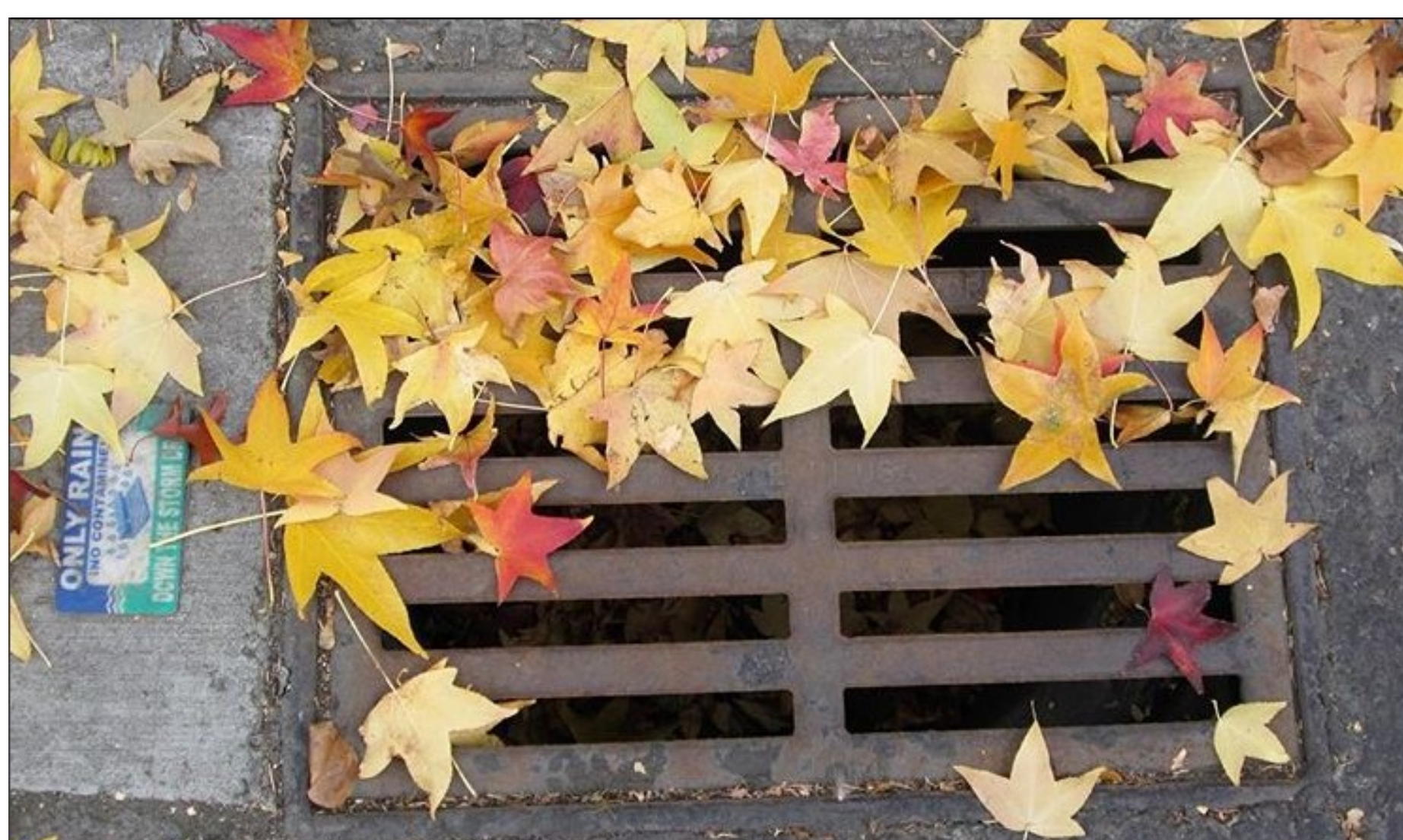
Yakima City Code forbids sweeping leaves and yard debris onto streets, gutters and sidewalks due to issues with leaves clogging storm drains.
