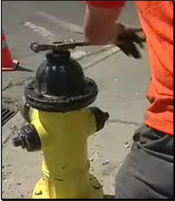
About 750 of the more than 3000 fire hydrants in Yakima are tested each year to ensure they are working properly.
