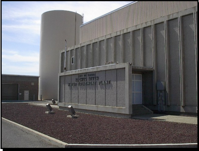
Yakima's drinking water treatment plant is located about 7 miles west of the city on Highway 12.
