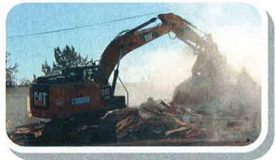
Tiger Mart at 24th and Nob Hill being demolished
