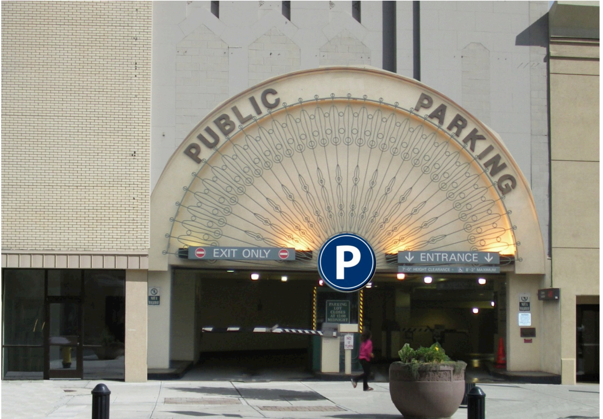
Mall Parking- Third Street Entry Ramp
