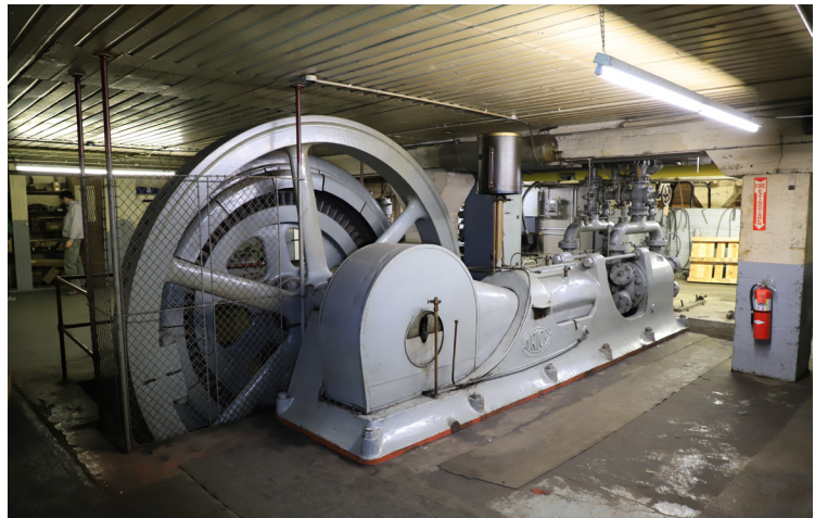
2019 view of an original ammonia compressor in the basement of the warehouse at 201 North 1st Avenue.
