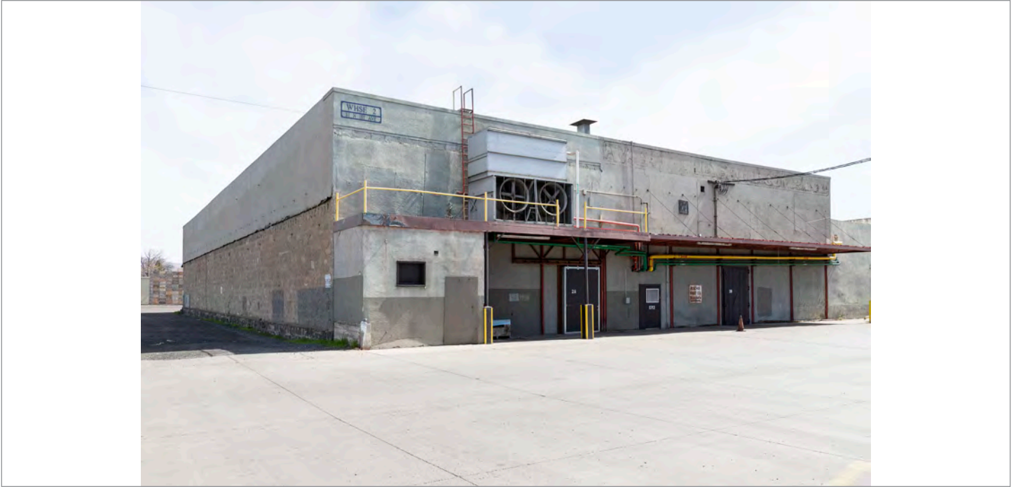
WA_Yakima County_Fruit Row_0041. Northwest corner of 313 N First Avenue.
