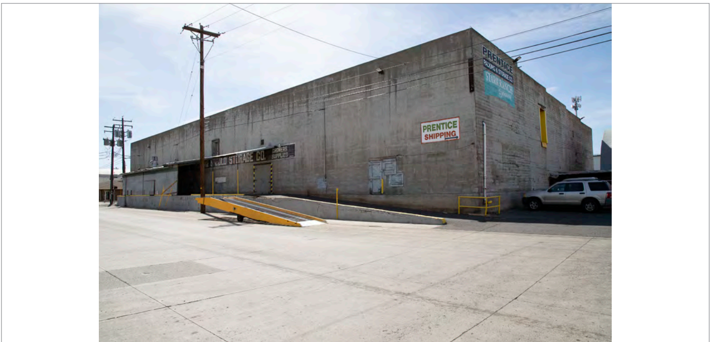
WA_Yakima County_Fruit Row_0022. Northeast corner of 202 N First Avenue.
