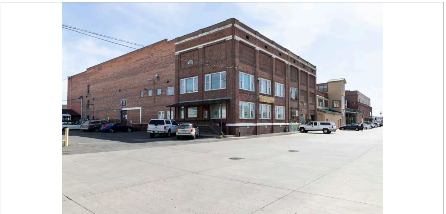
WA_Yakima County_Fruit Row_0008. Northwest corner of 29 N First Avenue.
