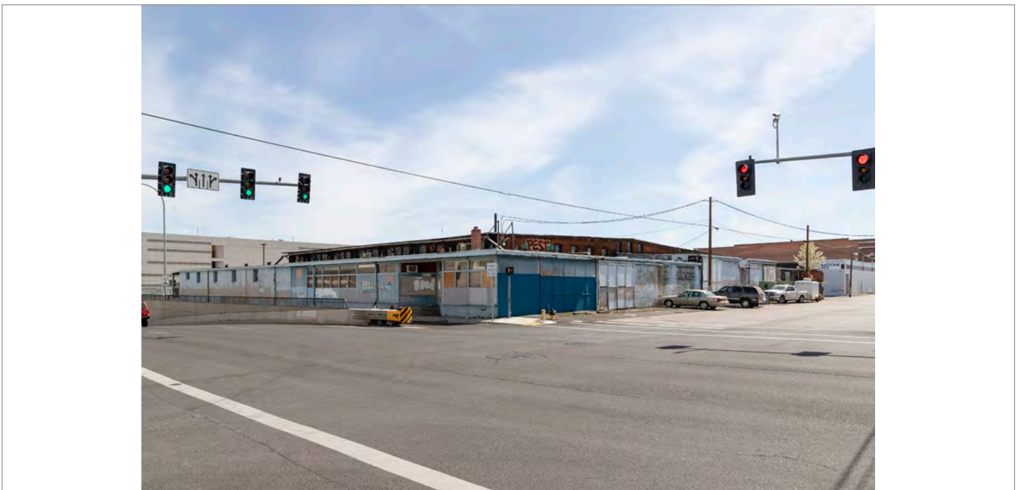
WA_Yakima County_Fruit Row_0016. Northwest corner of 117 N First Avenue.
