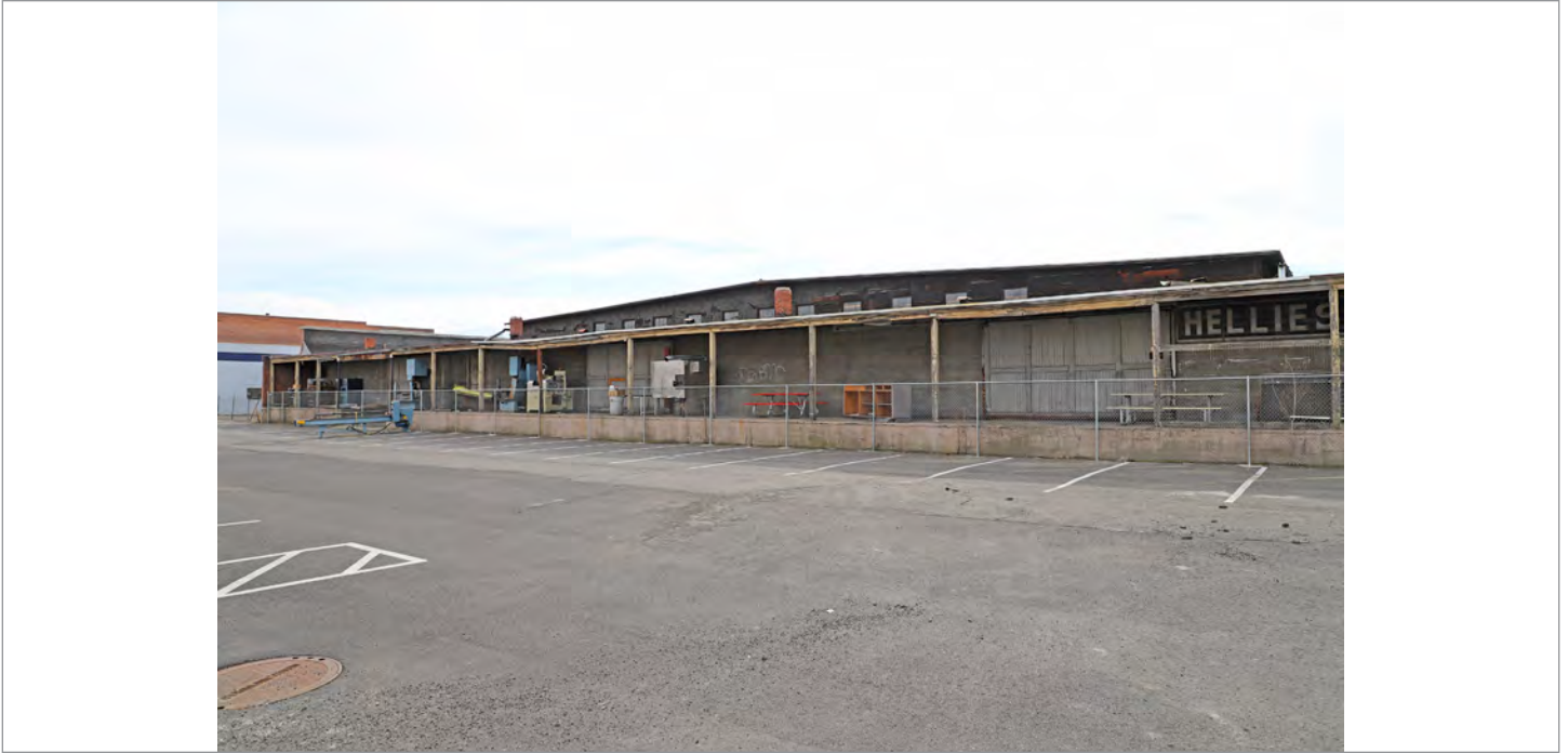
WA_Yakima County_Fruit Row_0017. Northeast corner of 117 N First Avenue.
