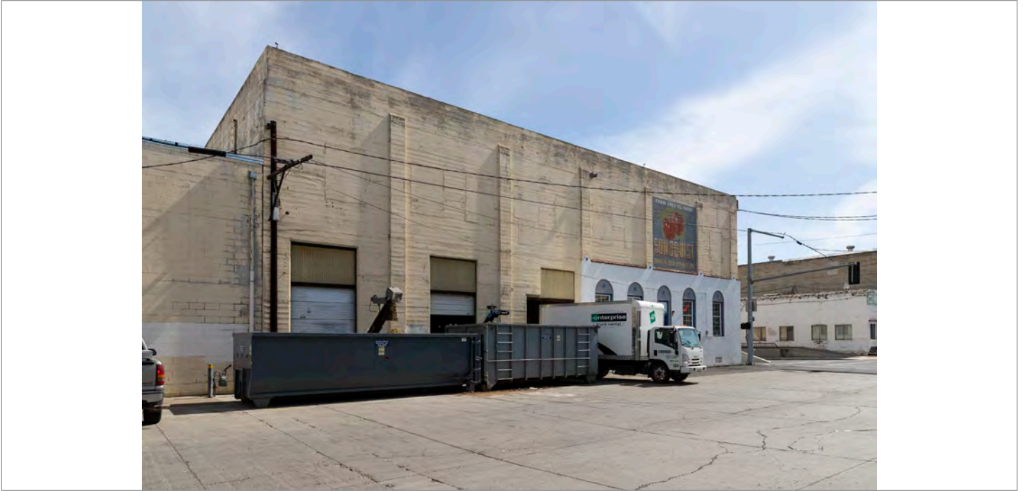
WA_Yakima County_Fruit Row_0035. Northwest corner of 301 N First Avenue.
