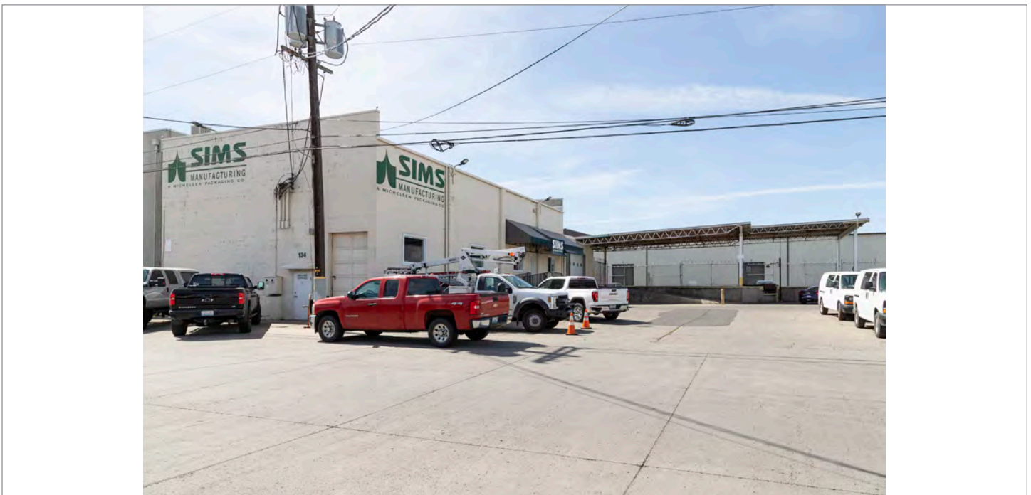
WA_Yakima County_Fruit Row_0014. Northeast corner of 134 First Avenue and the loading dock.
