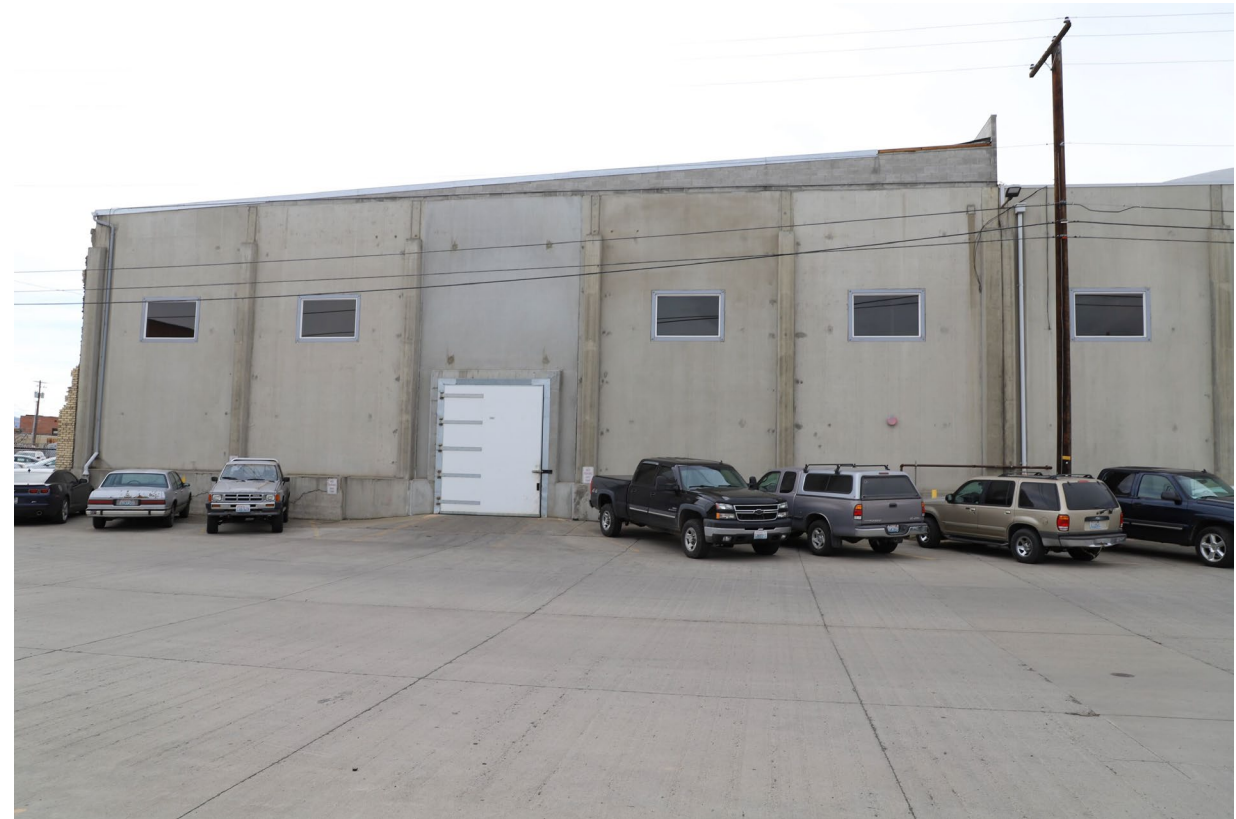
132 North First Avenue
