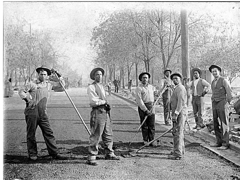
Road crew paving Naches Avenue, 1908.
