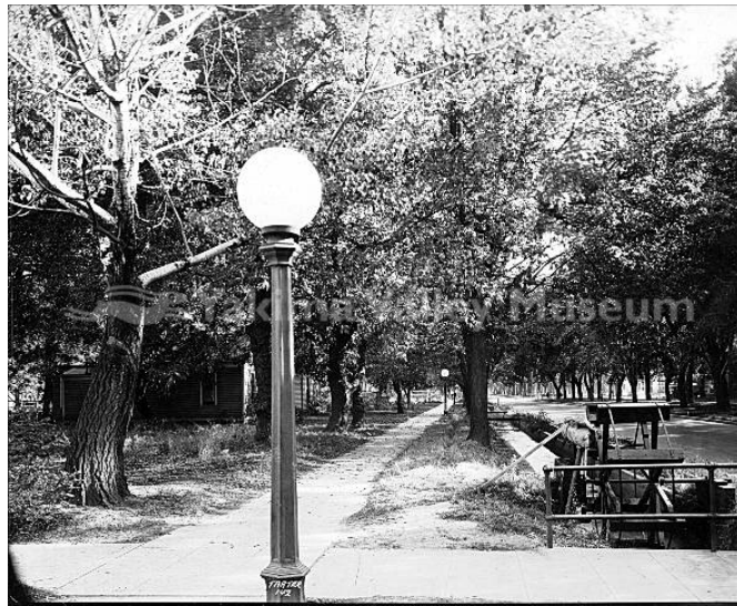
Naches Avenue, lighting standard and irrigation ditch, undated.
