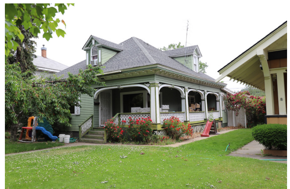
Figure 15. Hip Roof Example. 509 North Naches Avenue (ca. 1912), front southwest corner.
