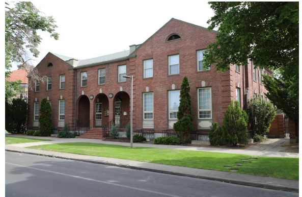
Figure 8. Facade Break Example. 15 North Naches Avenue (ca. 1934), front west facade showing the middle facade portion recess.
