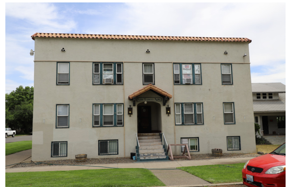
Figure 9. Low-rise Apartment Block Form Example. 415 North Naches Avenue (ca. 1925), front west facade.
