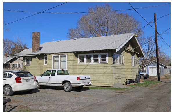
Figure 13. Wood Siding (Shingle) Example. 513B South Naches (ca. 1920), rear southeast corner along the alley.
