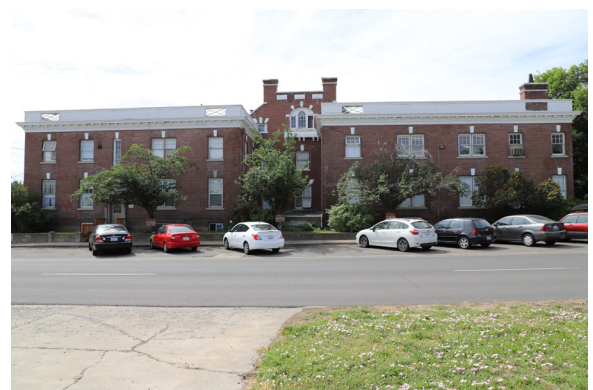
Figure 16. Flat with Parapet Roof Example. 115 North Naches (ca. 1930), side north facade.
