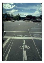
A pavement marking symbol that indicates the appropriate position for a bicycle to trigger a traffic signal.
