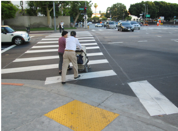
Not recommended: Diagonal curb ramp configuration.
