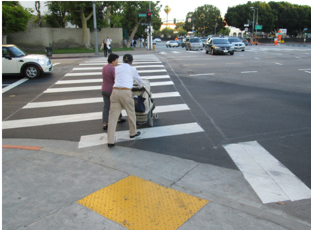
Not recommended: Diagonal curb ramp configuration.
