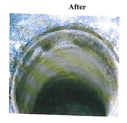
The City also has the ability to perform "cured in place pipe (CIPP) repair." This has allowed the City to complete needed work, without contracting it out. The CIPP process is useful for the permanent repair of cracks or voids in sewer pipes, effectively eliminating infiltration, all without having to excavate the pipe. In 2009, of the (9) repaired broken pipes, (4) were repaired utilizing the CIPP repair method.
