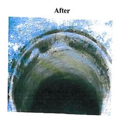
Another effective process conducted by the City is "cured in place pipe (CIPP) repair." This allows for the permanent repair of cracks or voids in sanitary sewer pipes eliminating infiltration, without having to excavate the pipe.
