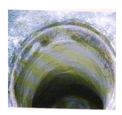
Also in 2005, the City purchased a bladder and repair kit in order to perform "cured in place pipe (CIPP) repair." Once again, allowing the City to complete the needed work, without contracting it out. The CIPP process is useful for the permanent repair of cracks or voids in sewer pipes, effectively eliminating infiltration, all without having to excavate the pipe. Since 2005, a total of 13 CIPP projects have been completed, 7 being completed in 2007 alone.
